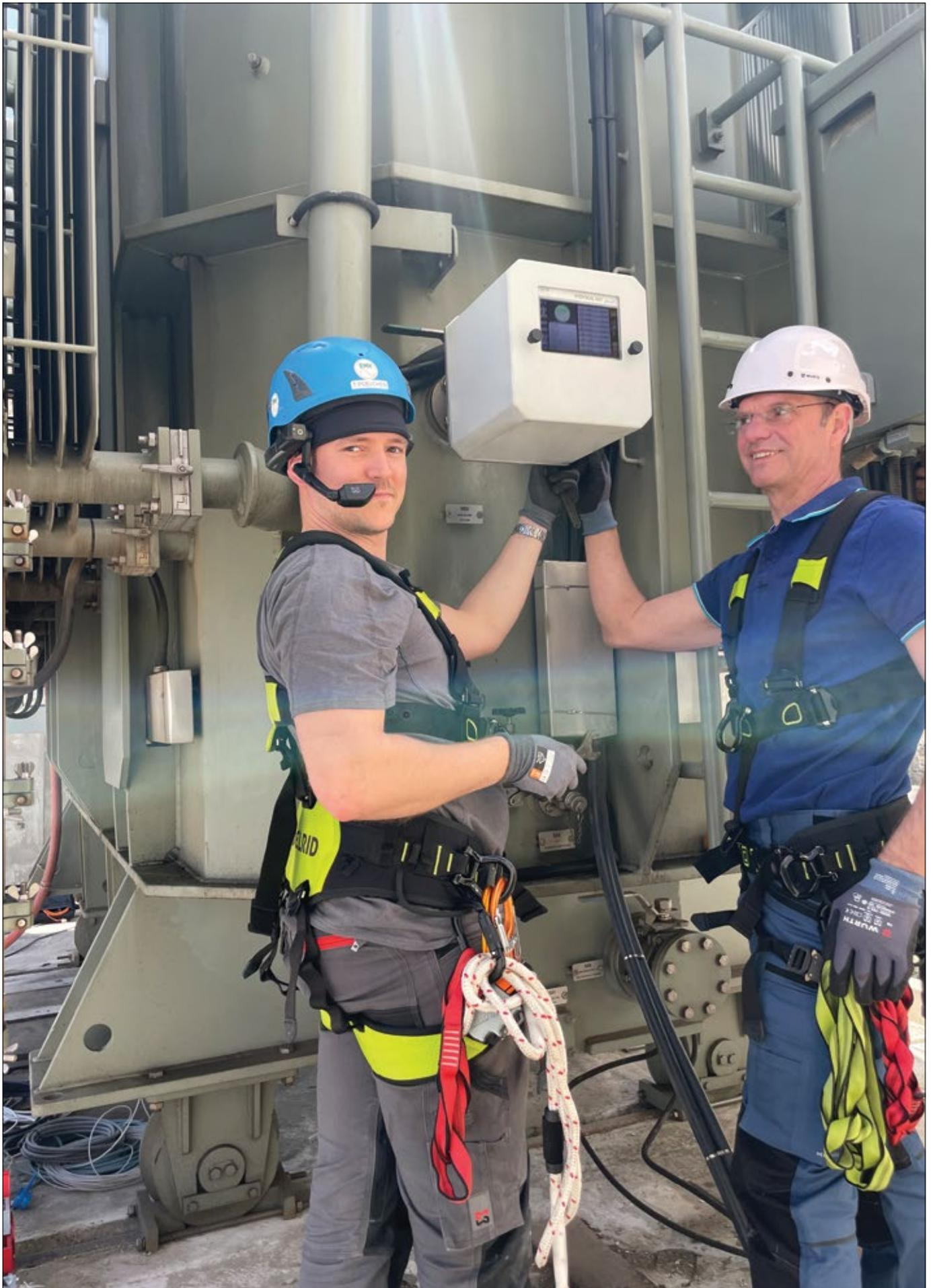
Figure 7. Successful commissioning of a HYDROCAL 1011 genX in the field
