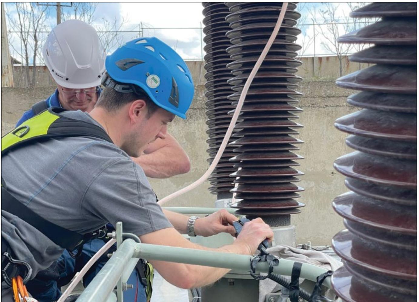
Figure 8. Installation of bushing sensors for the HYDROCAL BPD
